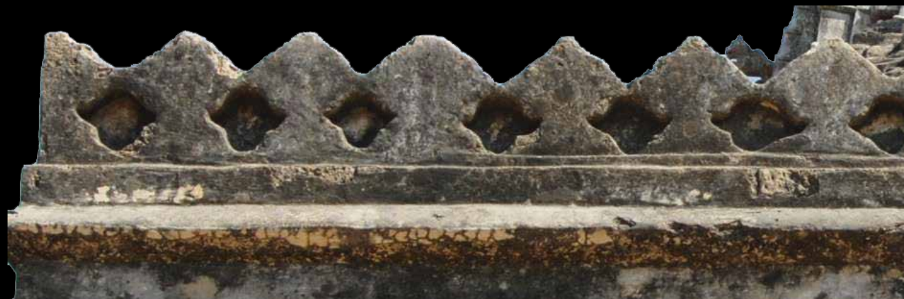
Figure 20. Merlons above the entrance wall
