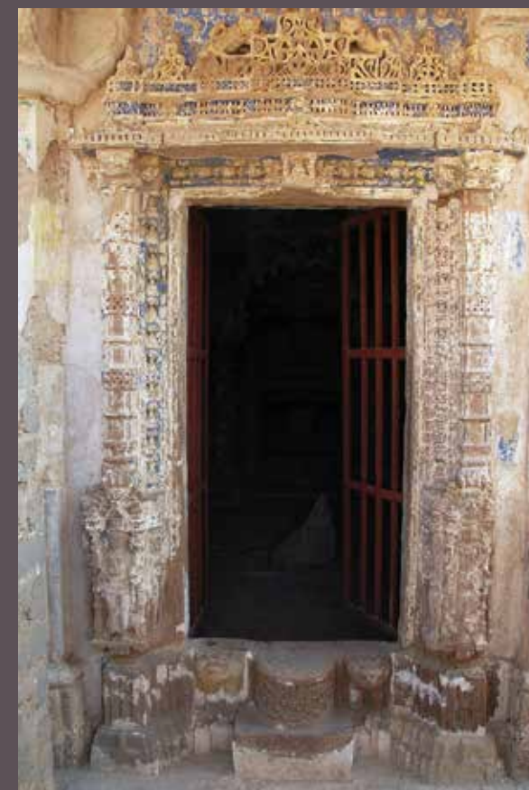
Figure 13. Door Frame of Mandapa
