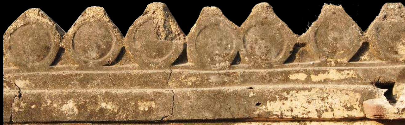
Figure 18. Merlons around Gambhara roof
